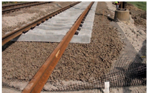
Base reinforcement for railway tracks
