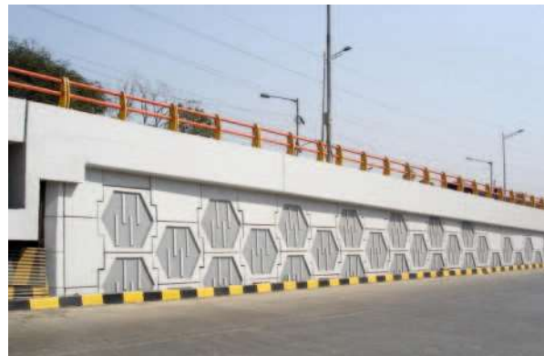
Reinforced Earth Wall
