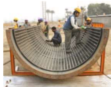
Adhesive application & Fixing
