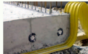
P.V.C. Water stop network at bottom of a water tank
